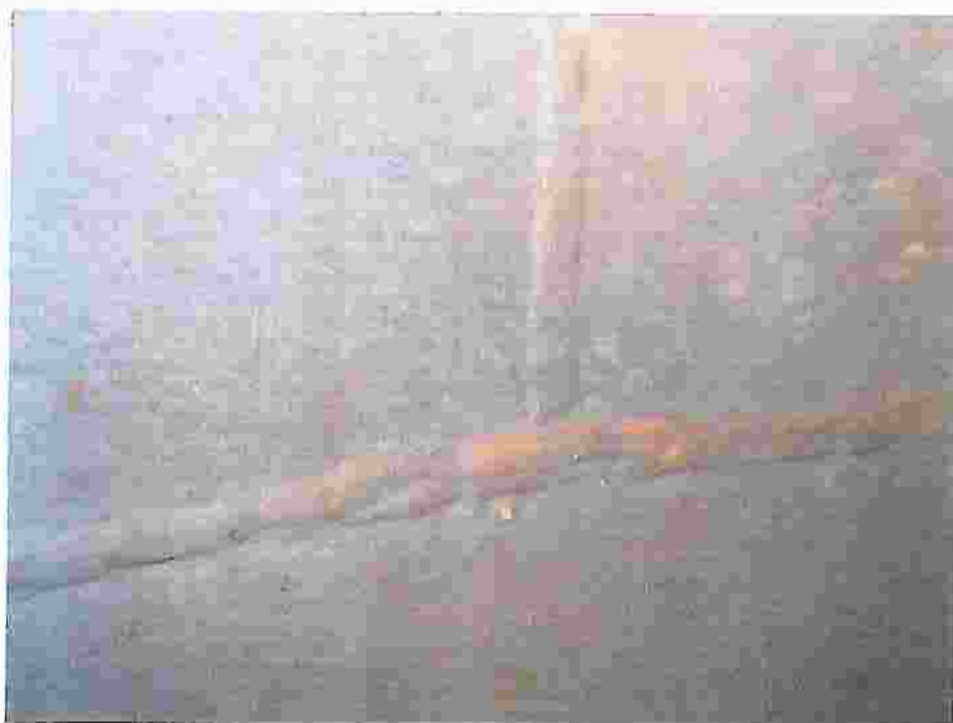
UPPER SHELL WELD SEAM; GOOD CONDITION
