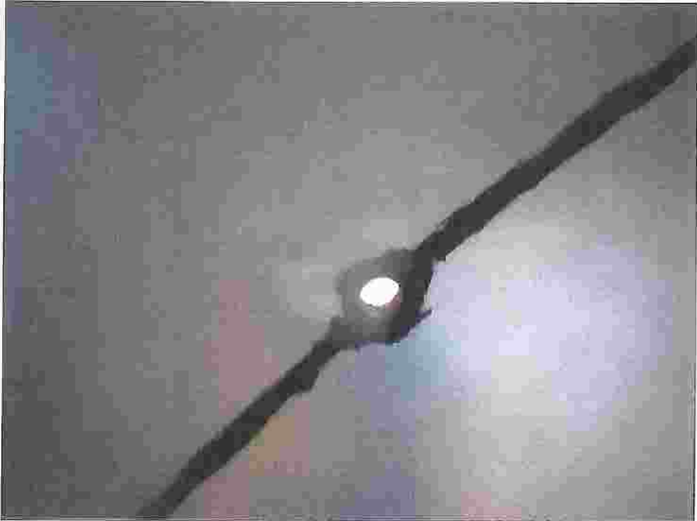
CEILING SURFACE WITH MASTIC COATING ON WELD SEAM
