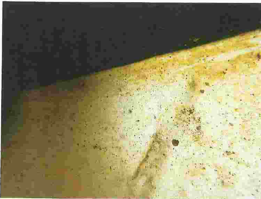
FLOOR/SHELL WELD SEAM
