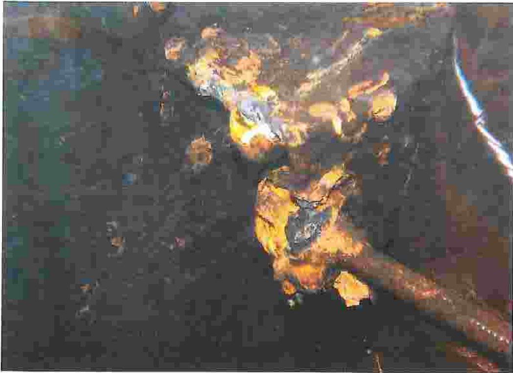
U-BOLT SECURING PVC TO SHELL
