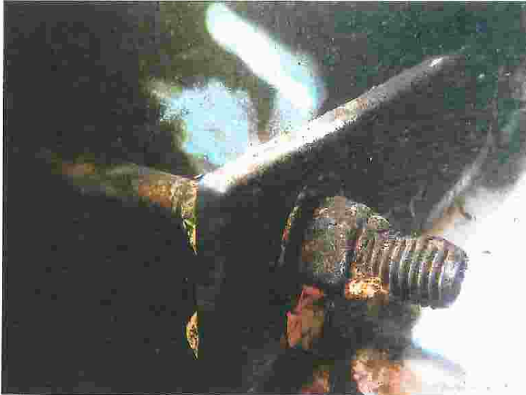
VERTICAL PVC SUPPORT BRACKET ON SHELL
